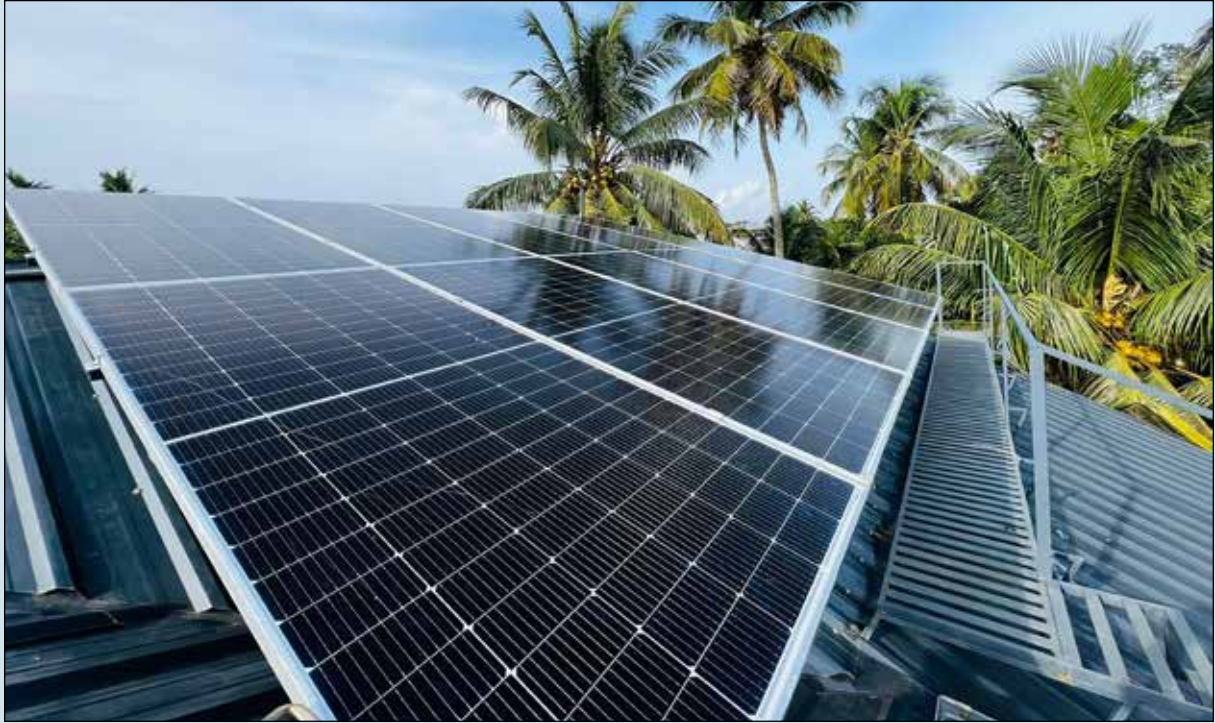
Top View of Solar Power plant Work at Kochi
